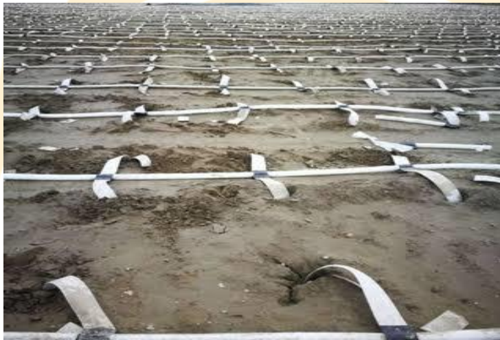
Fig: Installation Of PHD
