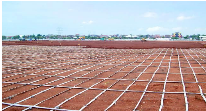
Fig: PHD (Prefabricated Horizontal Drain)
